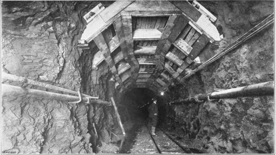
A completely dug-out and reinforced section of the tunnel below shaft 6 being prepared for concrete. 16th Annual Report of the Board of Water Supply (1/1/1922)
