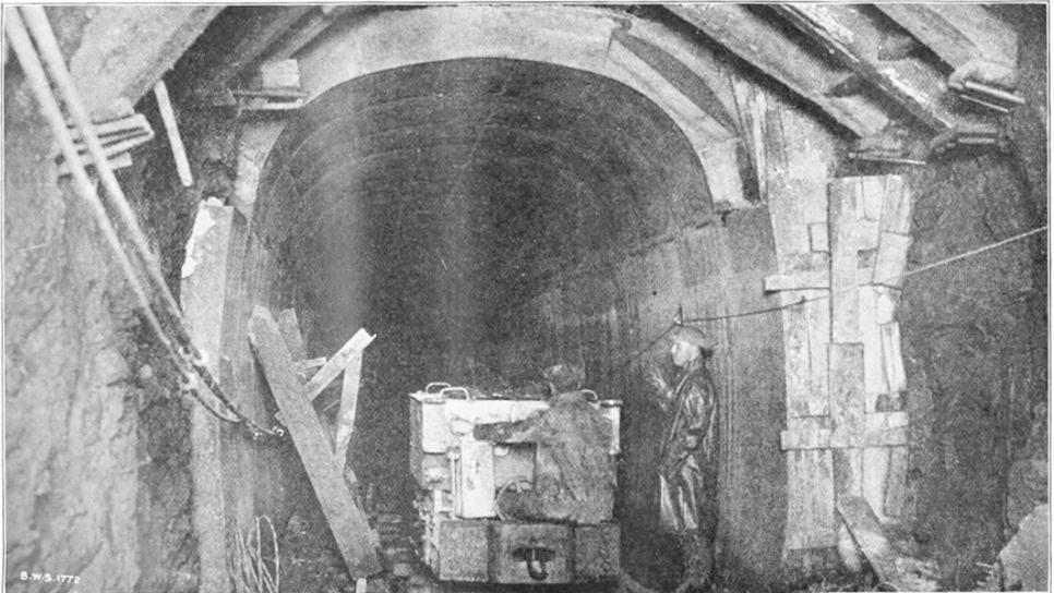
Concreted section of the tunnel about 700 feet south of shaft 5. This was the first portion of the Shandaken Tunnel completed. 17th Annual Report of the Board of Water Supply (1/1/1923)
