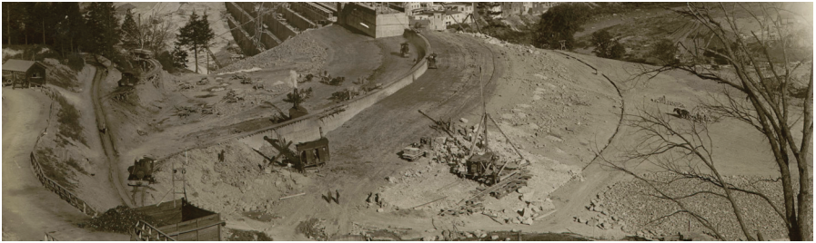
A sneak preview from 1925—a close-up of the berm just before the final backfill of dirt. Photo courtesy of the Department of Environmental Protection, Schoharie Reservoir, Gilboa Dam, Contract 203, Gilboa Division. Please do not distribute, reproduce or use these images for any other purpose without permission from DEP.
